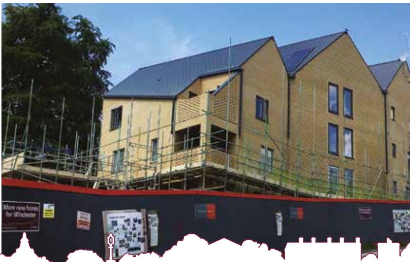
New homes under construction at The Valley, Stanmore
