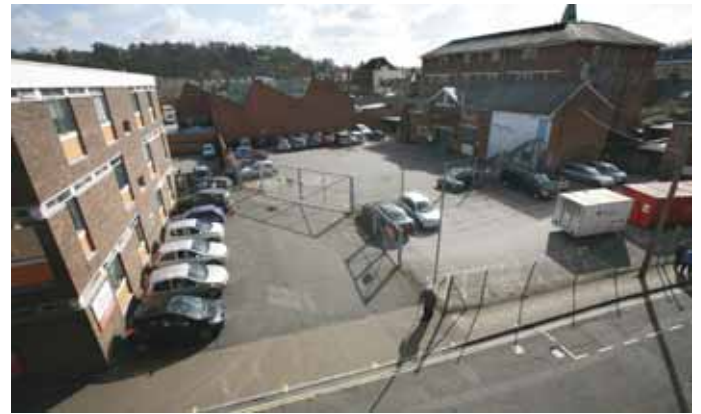
Silver Hill redevelopment site
