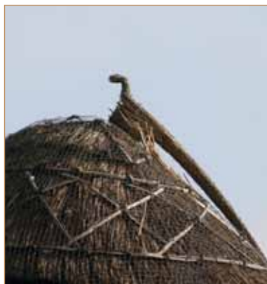
ornamental thatchwork at Compton End
