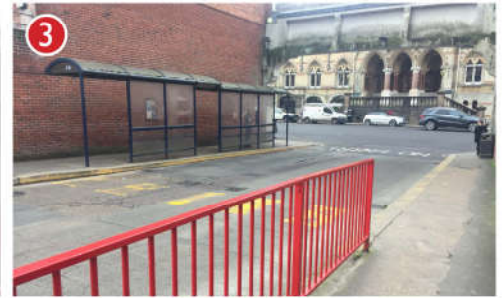
The bus station is not 'pedestrian friendly' with lengths of guardrail giving enclosed and narrow footways with no dropped kerbs or tactile paving.
