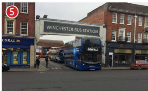
Buses leaving the bus station need to give way to vehicles on The Broadway and pull forward across the pedestrian desire line / footways.
