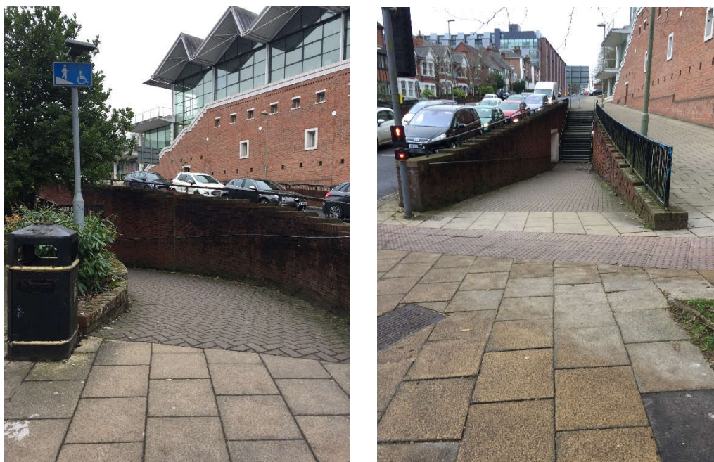
Figure 3-9 Pedestrian underpass on the B3420 South
