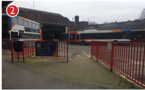
The bus station has a 'tired' and dated appearance.
