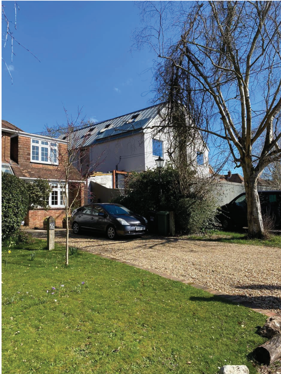
Appendix 1; Site photos taken by Officer 18 th March 2022
