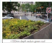
< 100mm depth sediment green roof
