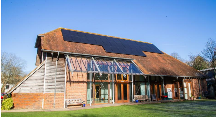
Itchen Abbas and Avington Village Hall, with an array of 36 solar panels, financed by LoCase and a successful local crowdfunding scheme
