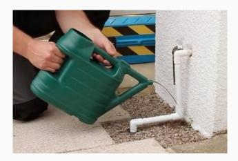
Frozen condensate pipes are one of the most common winter problems with modern boilers and, during very cold weather, the issue accounts for the highest percentage of repairs call outs. If part of your condensate pipework is outside, then in very cold weather it may freeze which could cause your boiler to stop working.
