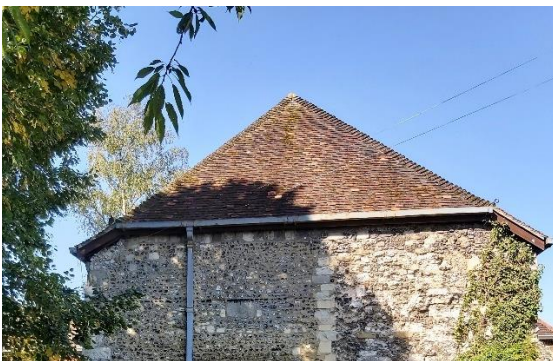
Fig 5 – View of east roof from ground level.
