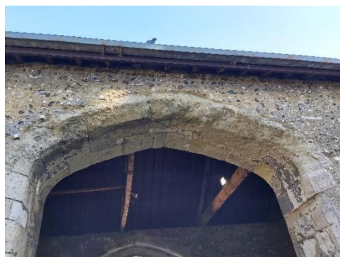
Fig 16 – Floodlights fixed to trusses in the carriageway.
