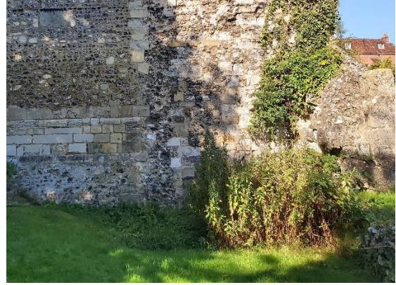
Fig 17 – Depression and wall heads to the east of the gateway.
