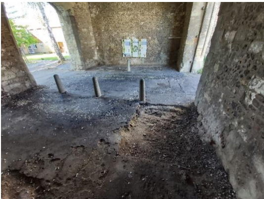
Fig 13 – Tarmac surfaces within the carriageway.
