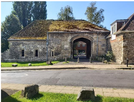
Fig 1 – The north elevation
