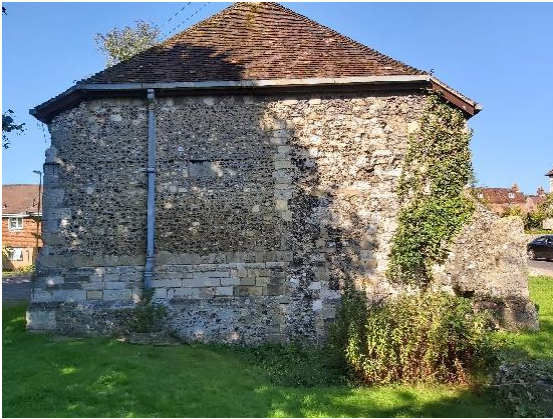
Fig 3 – The east elevation
