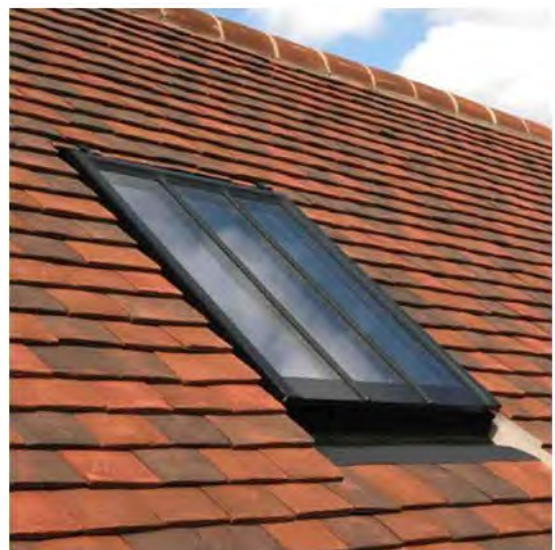
Photo 35. Conservation type skylight flush with roof surface.
