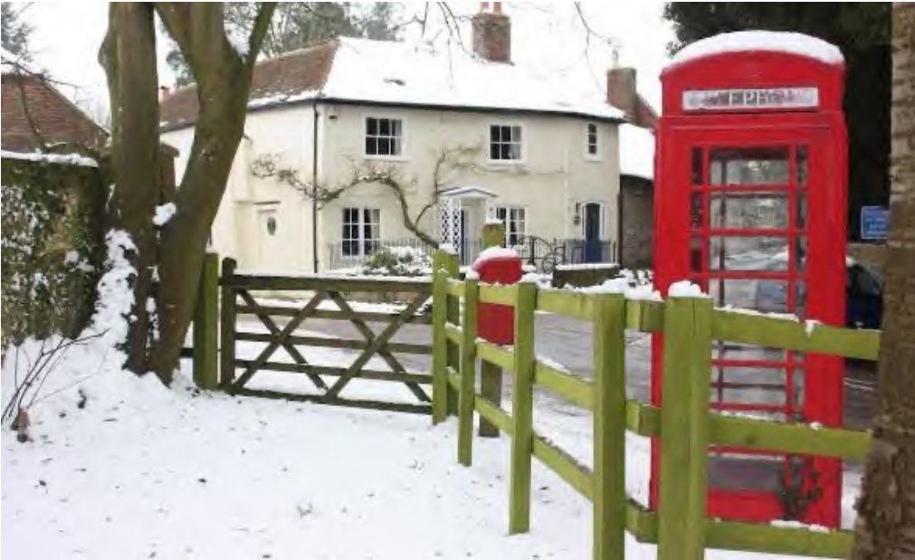
Photo 31. Pond House, Shoe Lane, with painted brickwork walls and former outbuilding in flint and red brick.
