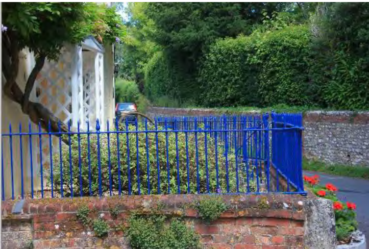
Photo 39. Simple painted metal railings at Pond House with brick and flint boundary wall beyond.
