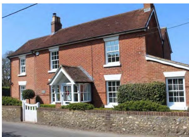
Photo 34. Sash windows with deep stone cill and frames set behind brickwork at Yew Tree Cottage
