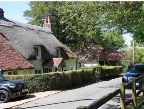
Photo 24. Little Croft on Church Street showing a variety of traditional building materials including thatch, clay plain roof and wall tiles, painted brick, and timber boarding.
