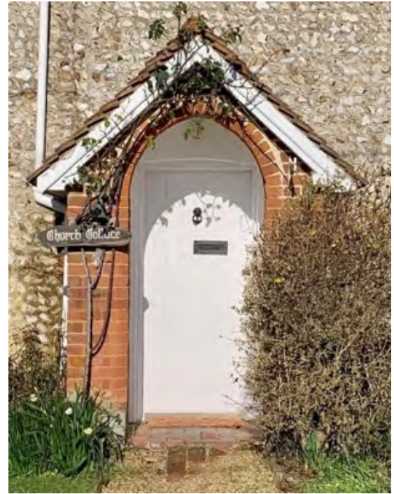
Photo 36, Porch at Church Cottage, Church Street.
