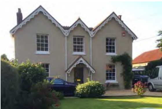
Photo 27. Gable ends facing the road are unusual in the village. The decorative barge boards are also not typical but add to the visual variety in the street.
