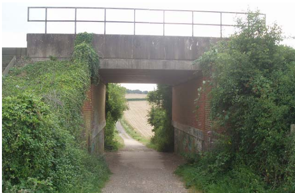
Bridge carrying the main line railway at Barton Farm
