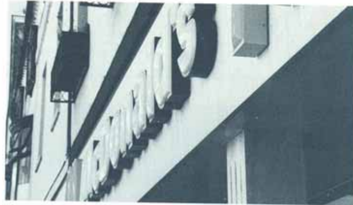
Inappropriate mounted plastic lettering can appear out of place when on an older building.
