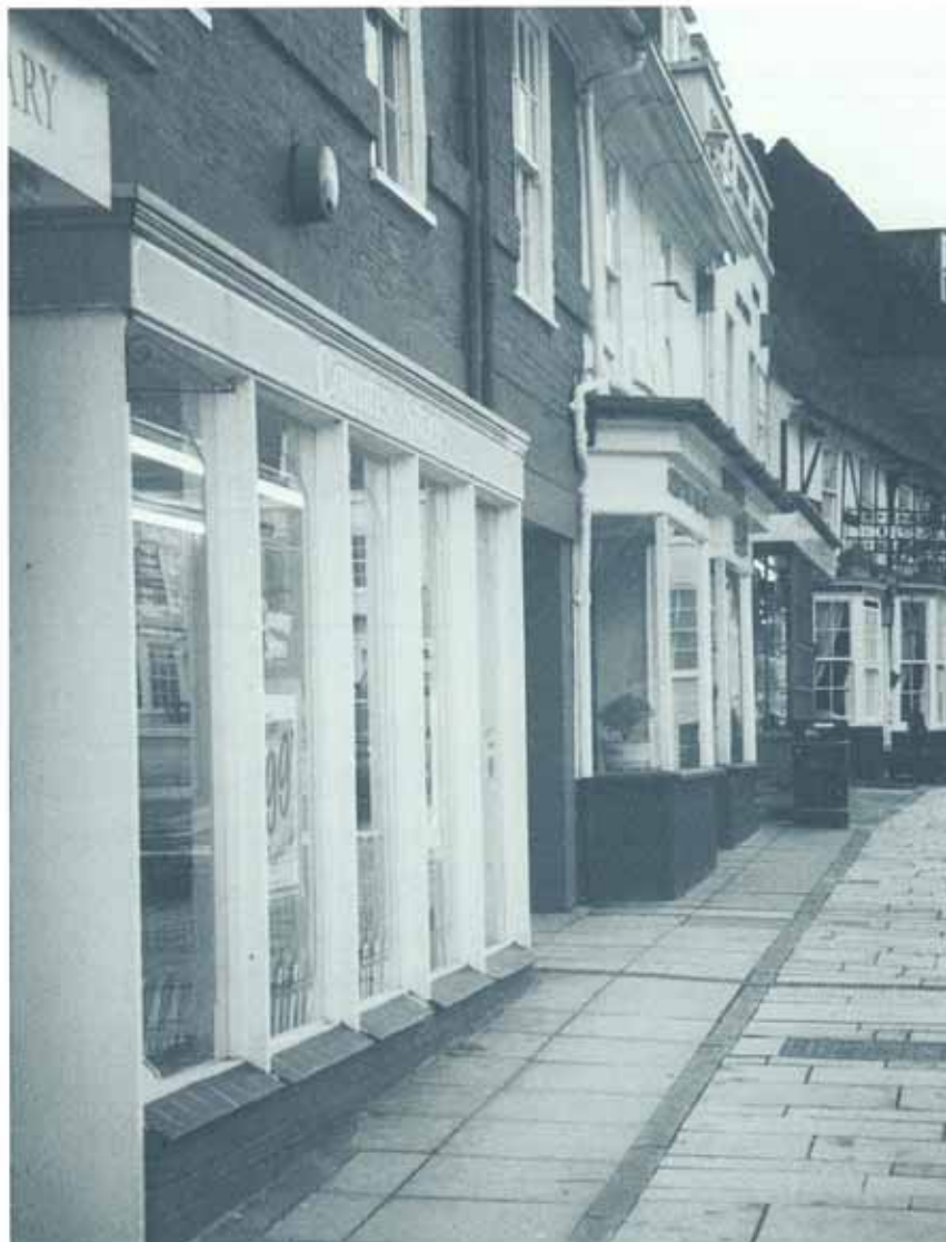
Use of deep mullions minimising visual clutter of advertising, County Stores Broad Street Alresford
