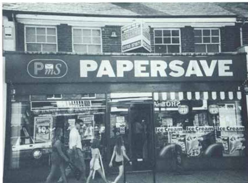
Lettering that is out of scale, together with excessive stick-on signs, results in a design that obscures the visibility of the building and the inside of the shopfront.
