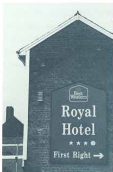
In certain instances, it may be acceptable to mount advanced warning signs on walls, which overcomes the problems of safety and visual clutter at street level.
