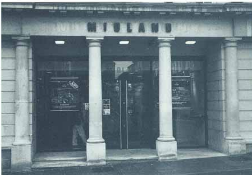
Use of Lobby Bank, Midland Bank, High Street Winchester
